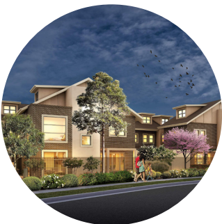
281-283 Peats Ferry Road, Hornsby
